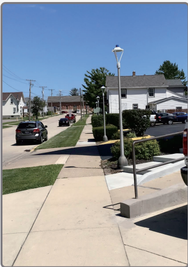
Street scapes lighting
