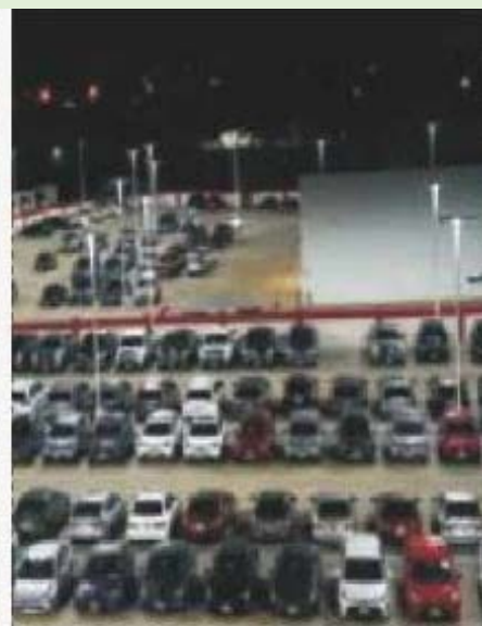
Parking lot Lighting
